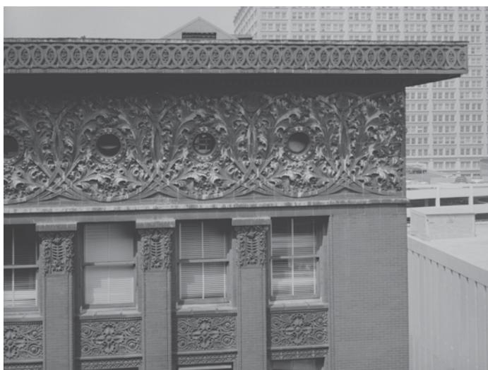
Wainwright Building, designed by Louis Sullivan, constructed 1890–1891. Historic American Building Survey, Library of Congress.
